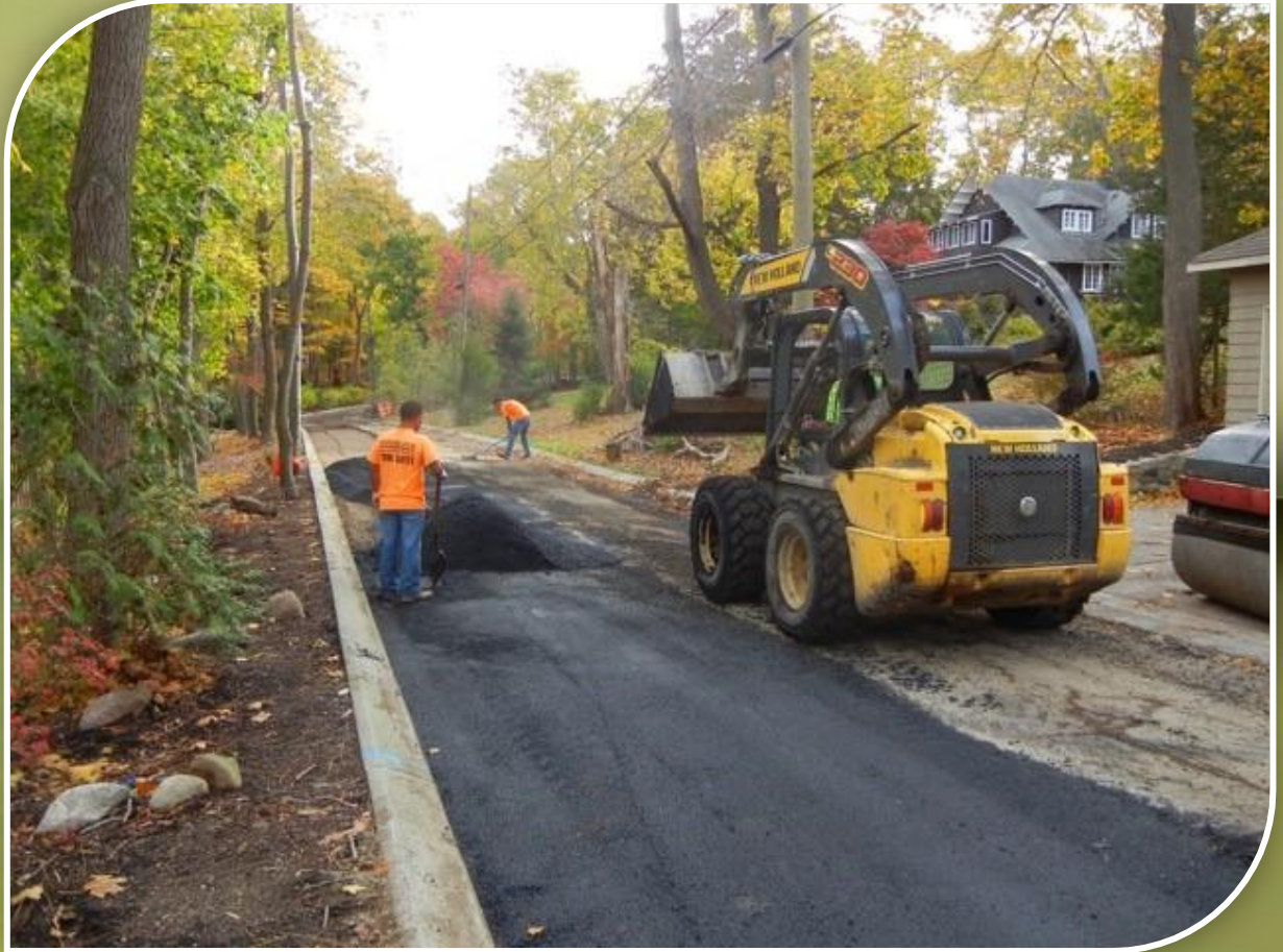
Tagliabue, first layer of asphalt
